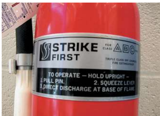
Figure1- 5 A typical fire extinguisher designed to be used on type class A, B, or C fires.
