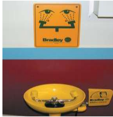
Figure1- 8 A typical eye wash station. Often a thorough flushing of the eyes with water is the best treatment in the event of eye contamination.
